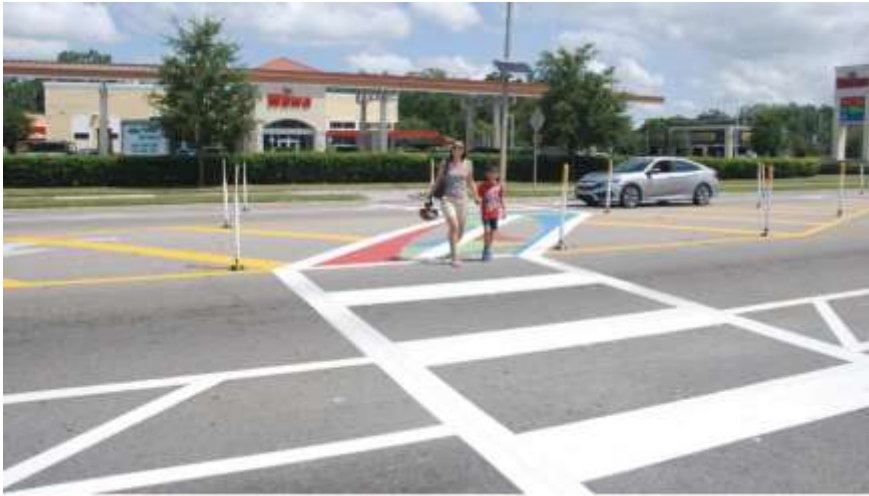
Orlando's demonstration project on Curry Ford Road added a new mid-block crossing with a painted, protected pedestrian refuge.
