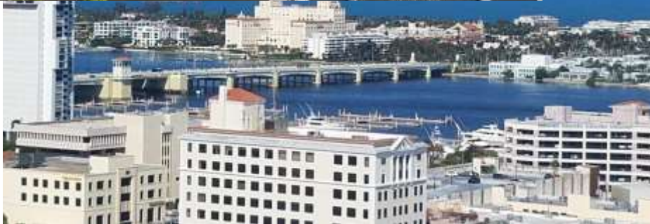
Flagler Bridge Replacement
