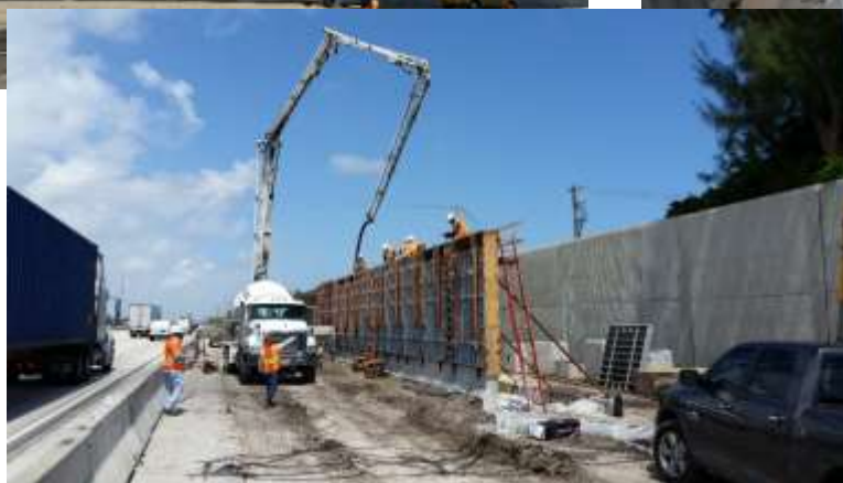
New interchange at I-95 at Spanish River
