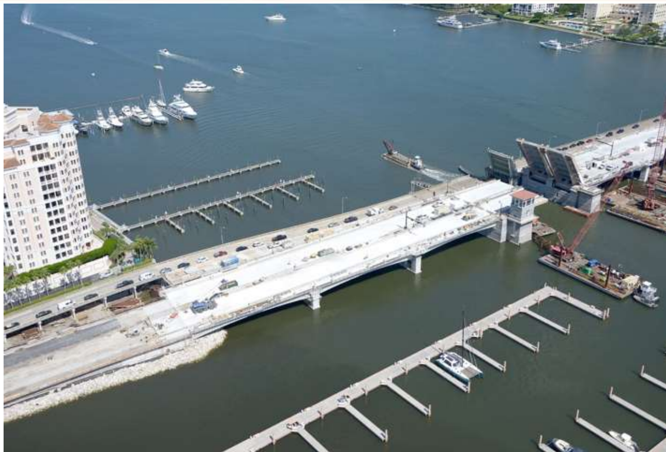
Flagler Bridge Replacement
