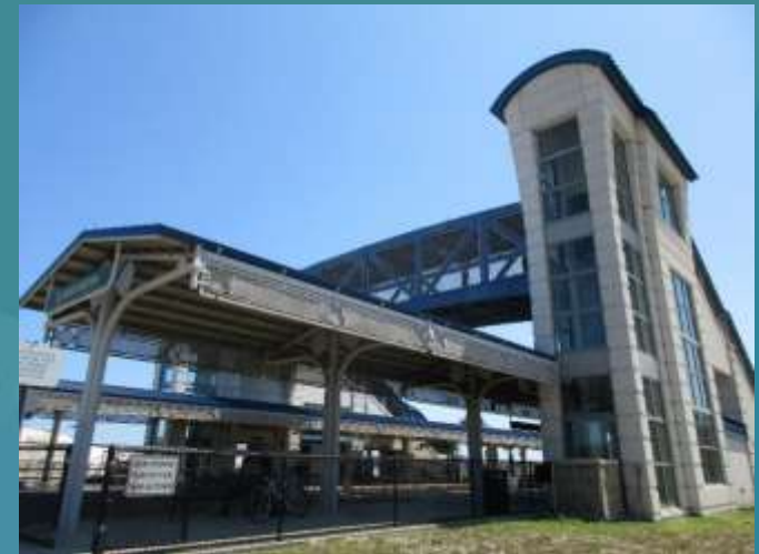
Existing Boca Raton Tri-Rail Station at Yamato Road
