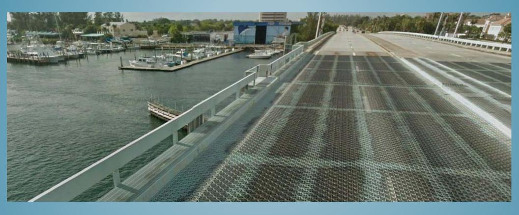
Movable Span Has Open Grid Deck
