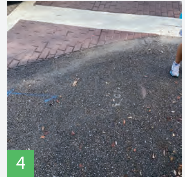
4 Install detectable warning at curb ramp
