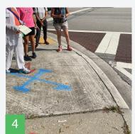
Extend the curb radii to create a bulb out
